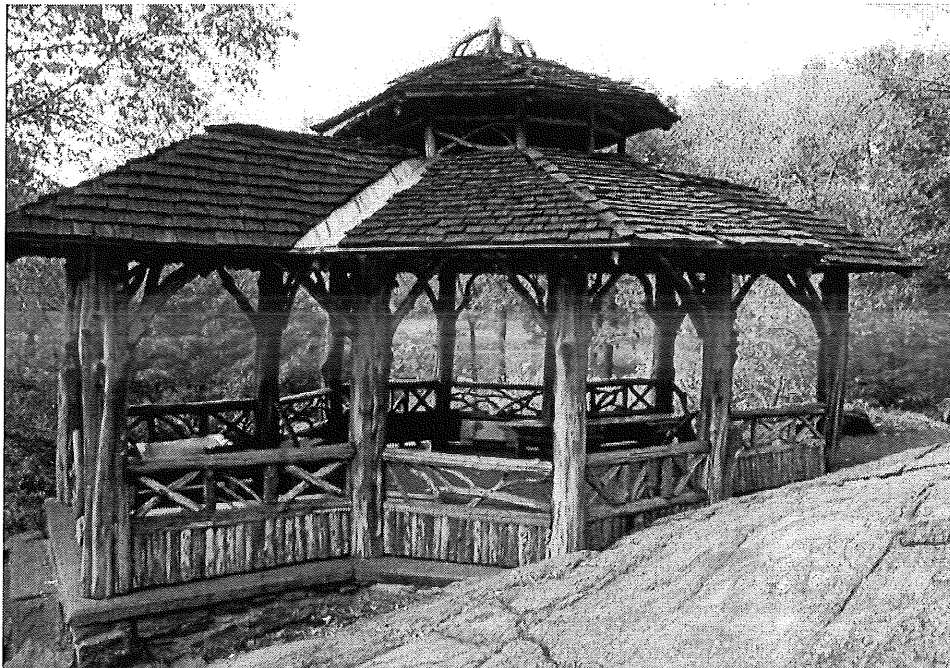
Rustic Small Shelter, Central Park, NY
