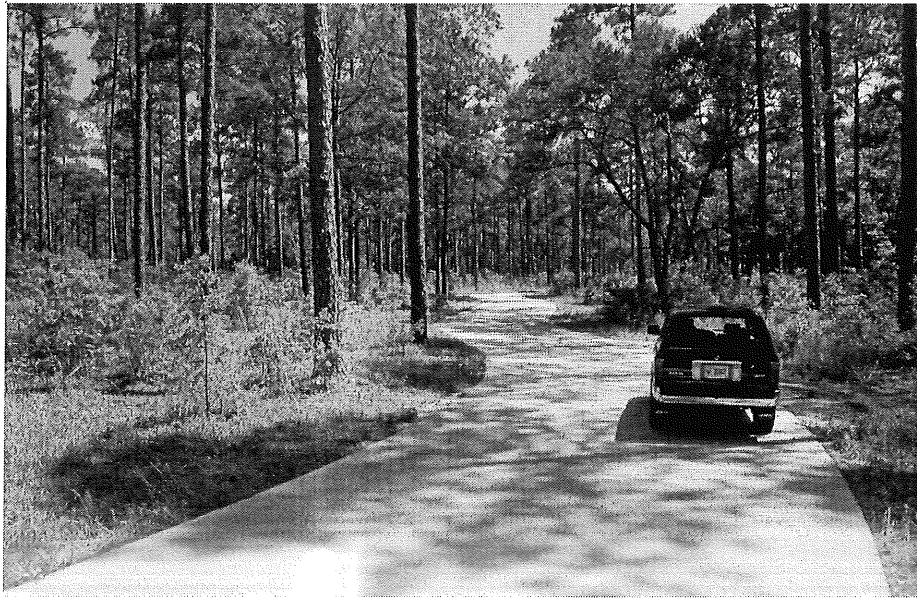
Pervious Concrete Driveway, Joseph W. Jones Ecological Research Center
